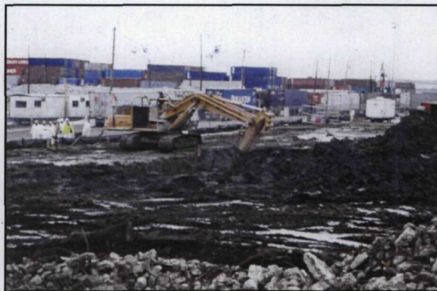
Figure 2. In situ S/S treatment at a former wood preserving facility in Port Newark, NJ.
