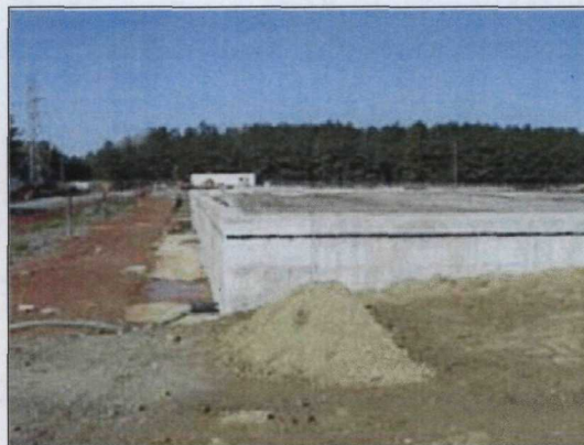
Construction of "divider wall" at the Rentokil site. All development must occur within the walls to prevent cover disruption.
