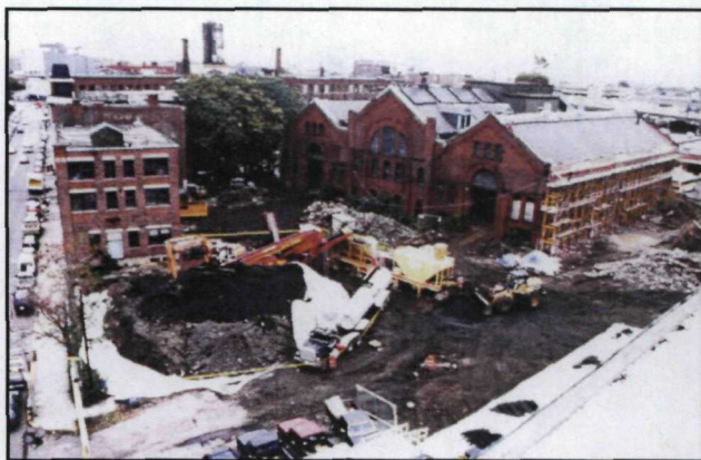
Figure 5. Ex situ S/S treatment of lead- and arsenic-contaminated soils in Boston, MA.
